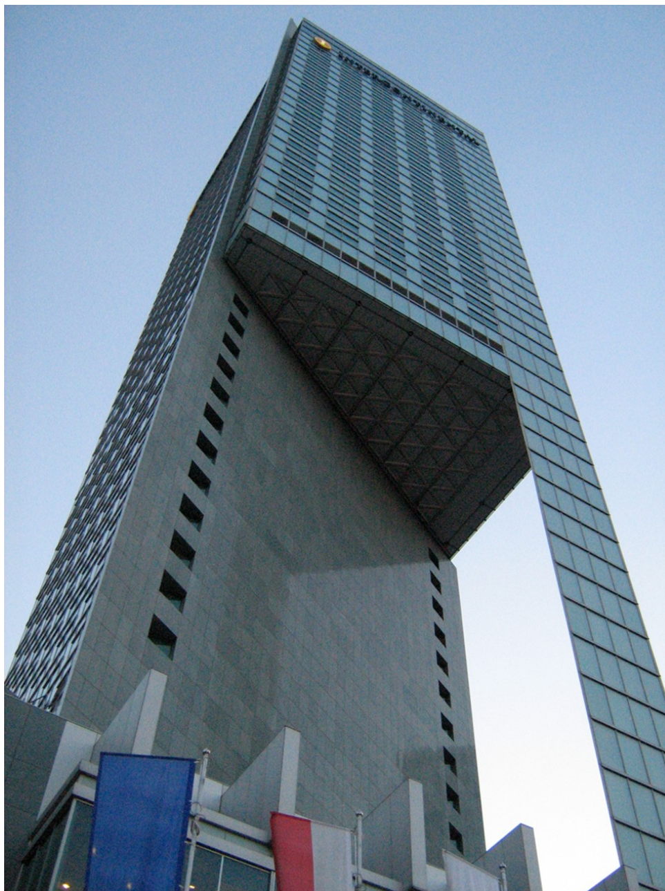
Intercontinental Hotel in Warsaw
