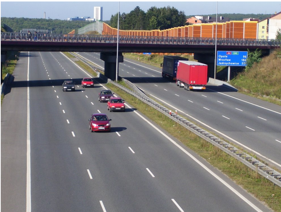
A4 motorway bridge in Ruda Śląska-Kochłowice
